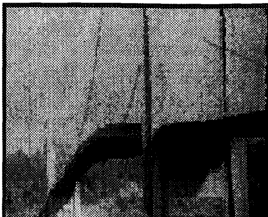
Fig. 1. Tacoma Narrows bridge in oscillation.
