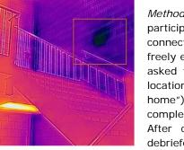
**Figure 5:** A participant in our pilot study surveyed a campus building and noticed an anomalous signature (center of red boxes) in an exterior wall that they could not explain. It was suggested, by other occupants of the building, that this was the site of a previous repair and that perhaps the wall was not restored to its previous condition.
