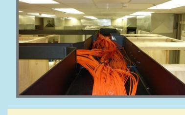
Figure 4: The optical cables connecting groups
